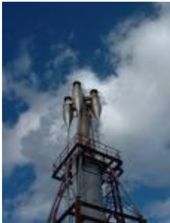
Energy - Wasted steam
