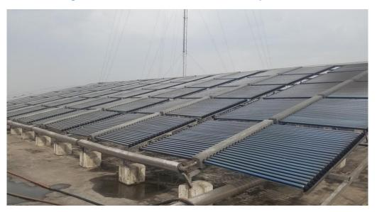
Figure 9: Solar water heater installed at a roof-top in Pakistan
