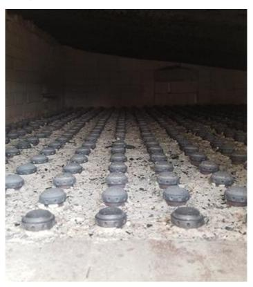
Figure 2: Combustion chamber of fluidized bed boiler
