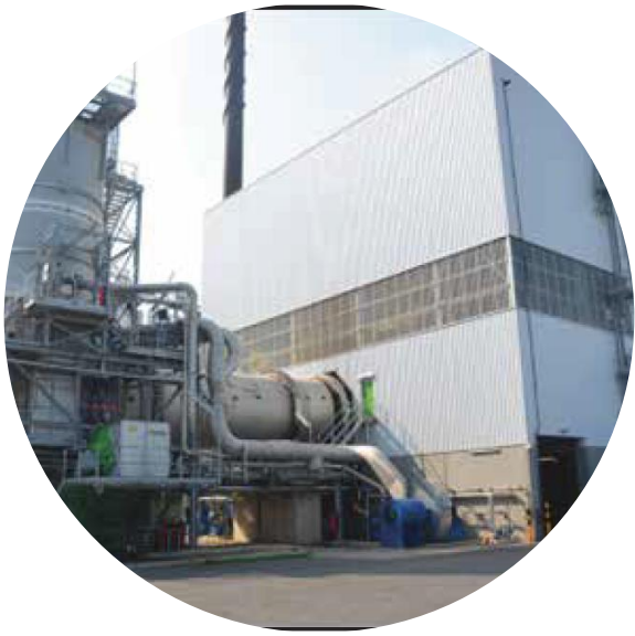
Sludge incinerator
