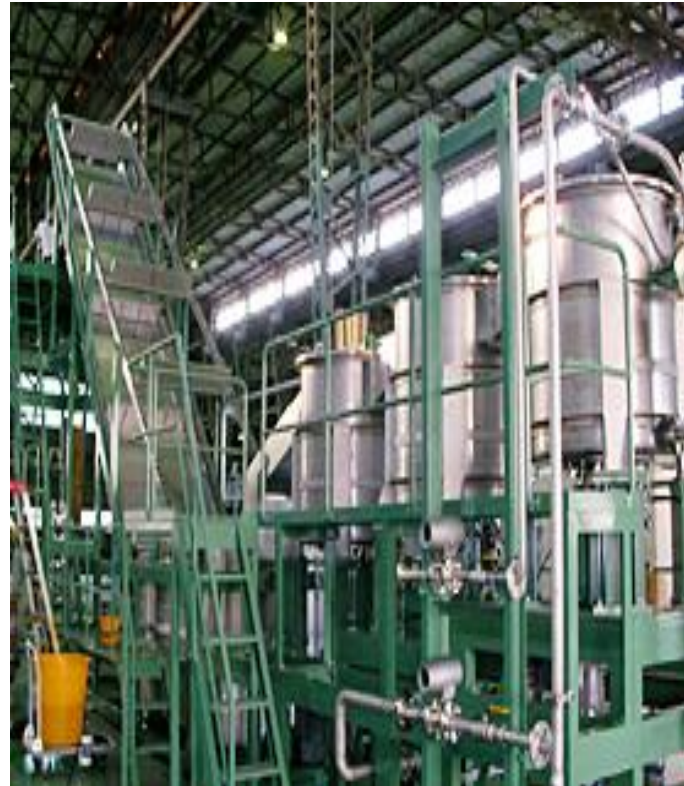
PVA Recovery Plant
